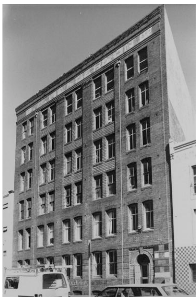
Figure 5.3.10 Former Henderson factory in 1978
