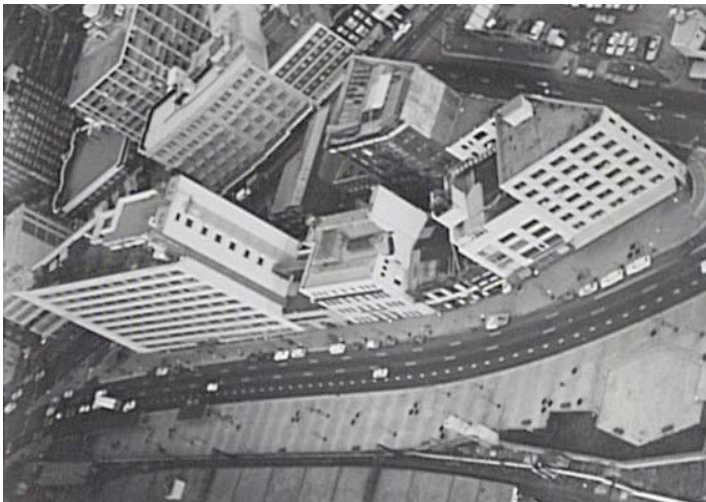
View to the sites in 978 Randle Street in 1989 – City of Sydney Archives SRC 4368
